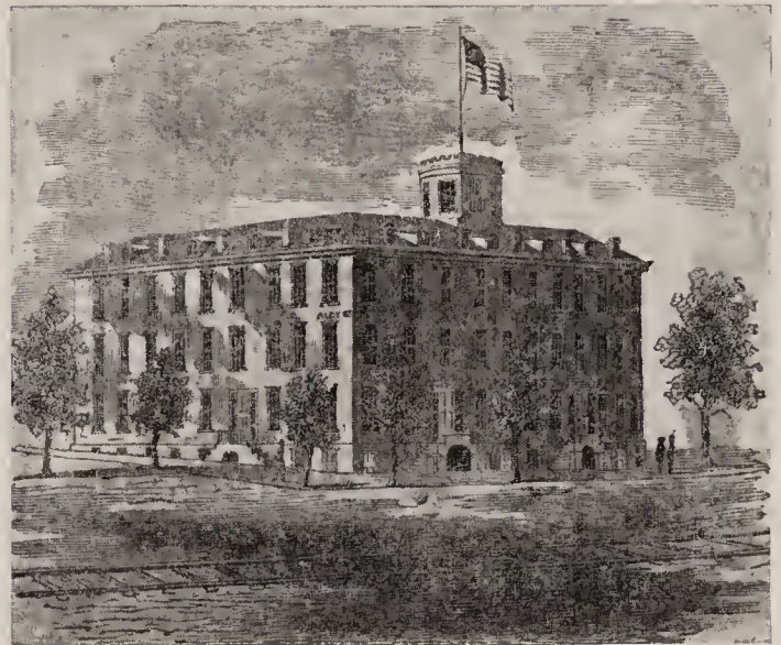
ALTON HOUSE, WHERE DOUGLAS STOPPED
